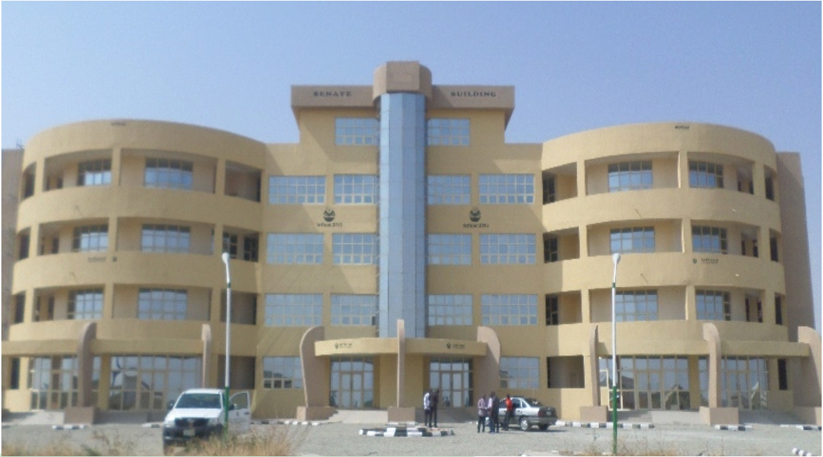
Construction of Senate Building, Bauchi State University, Gadau, Bauchi State.
