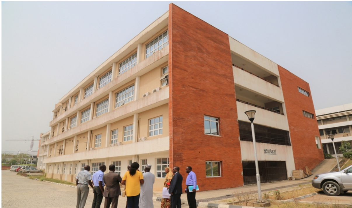
Pharmacy Phase II Building, Obafemi Awolowo University, Ile-Ife
