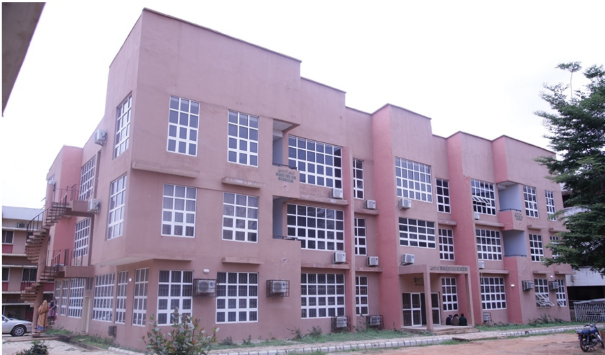
Staff Offices and Complex for College of Science and Technology, Kaduna State University
