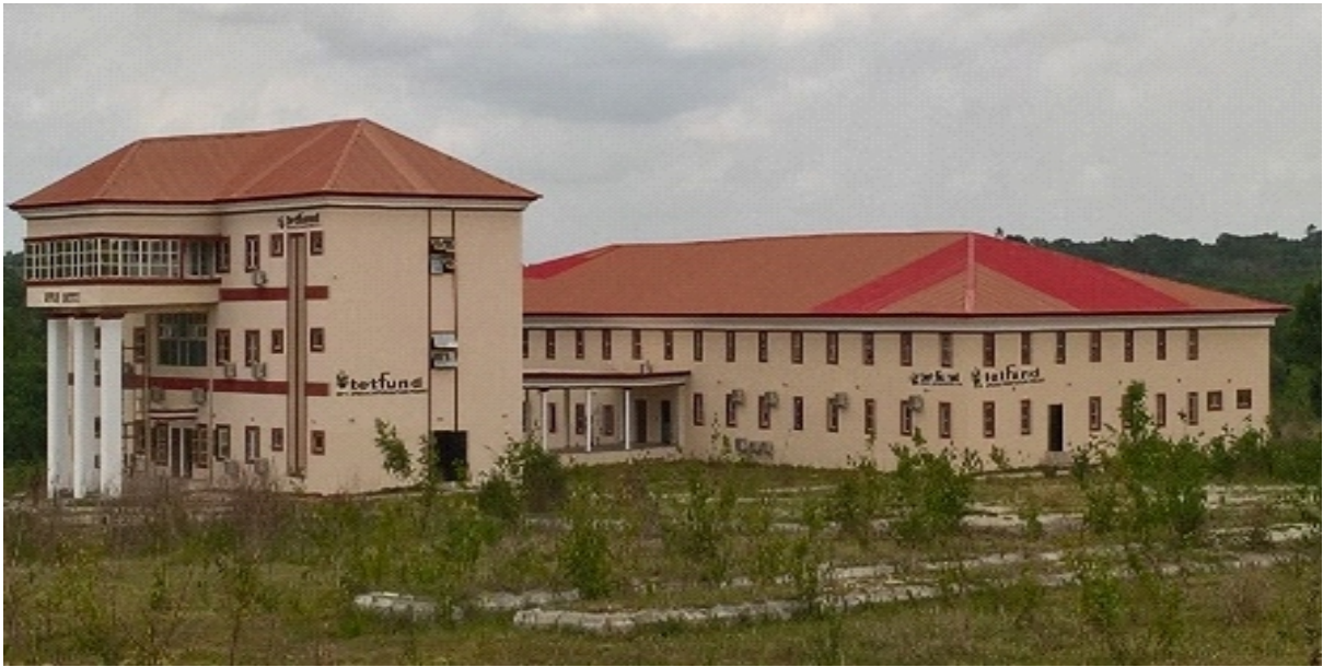
Construction and Furnishing of Software Institute, Ladoke Akintola University Ogbomosho, Oyo State
