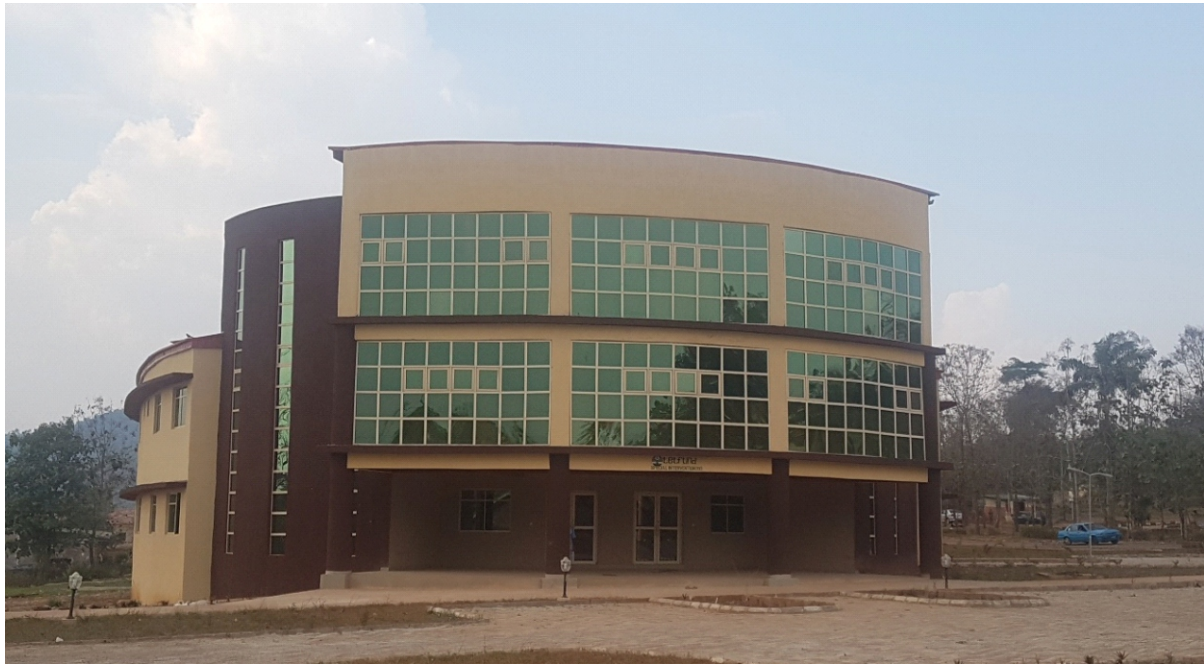
Construction of Two Storey Staff Academic Building, Osun State College Of Education, Ilesha
