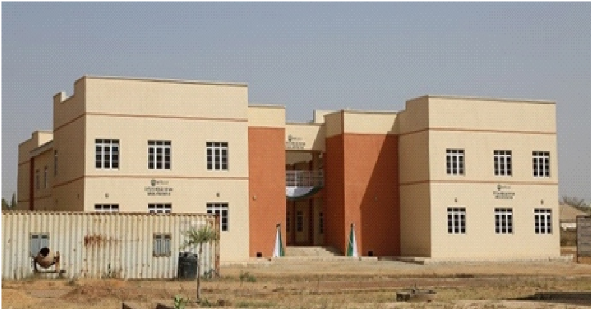
18 Classroom Block Lecture Hall, Abubakar Tatari Ali Polytechnic, Bauchi
