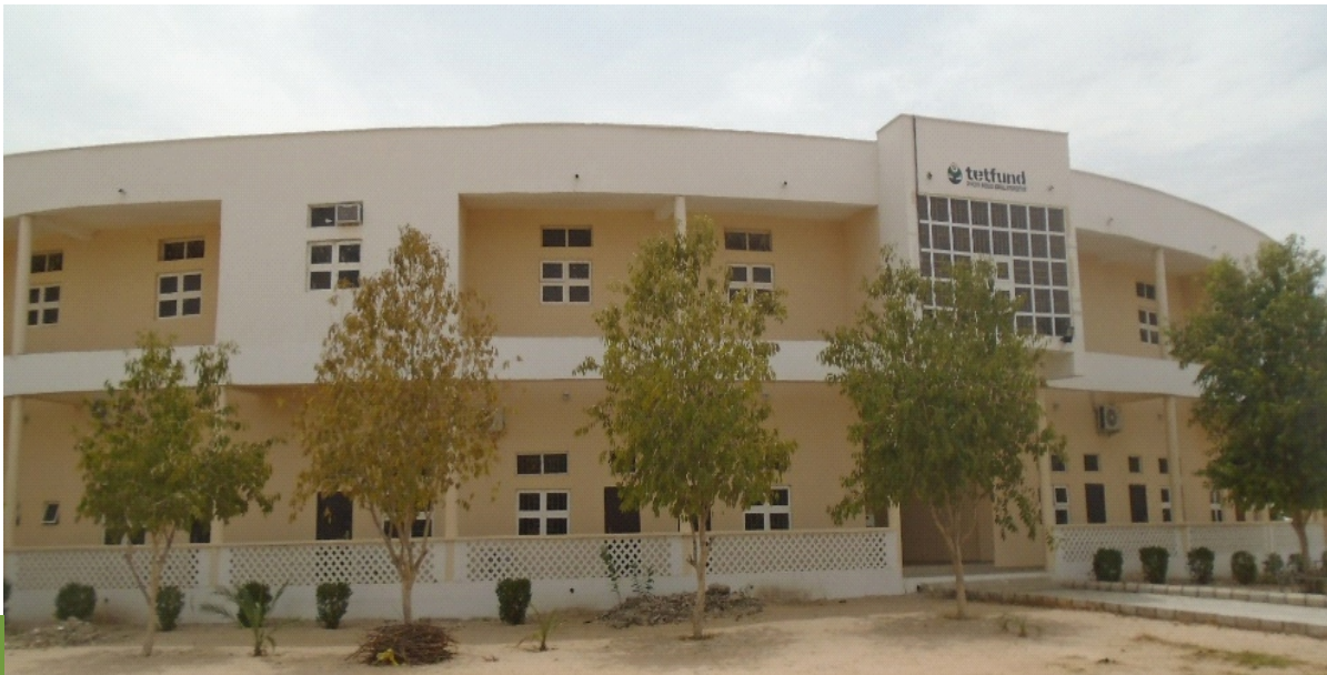
Rehabilitation of 1000- Capacity Auditorium, University of Maiduguri
