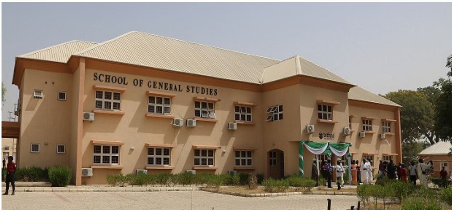
School of General Studies Building, Federal Polytechnic, Bauchi
