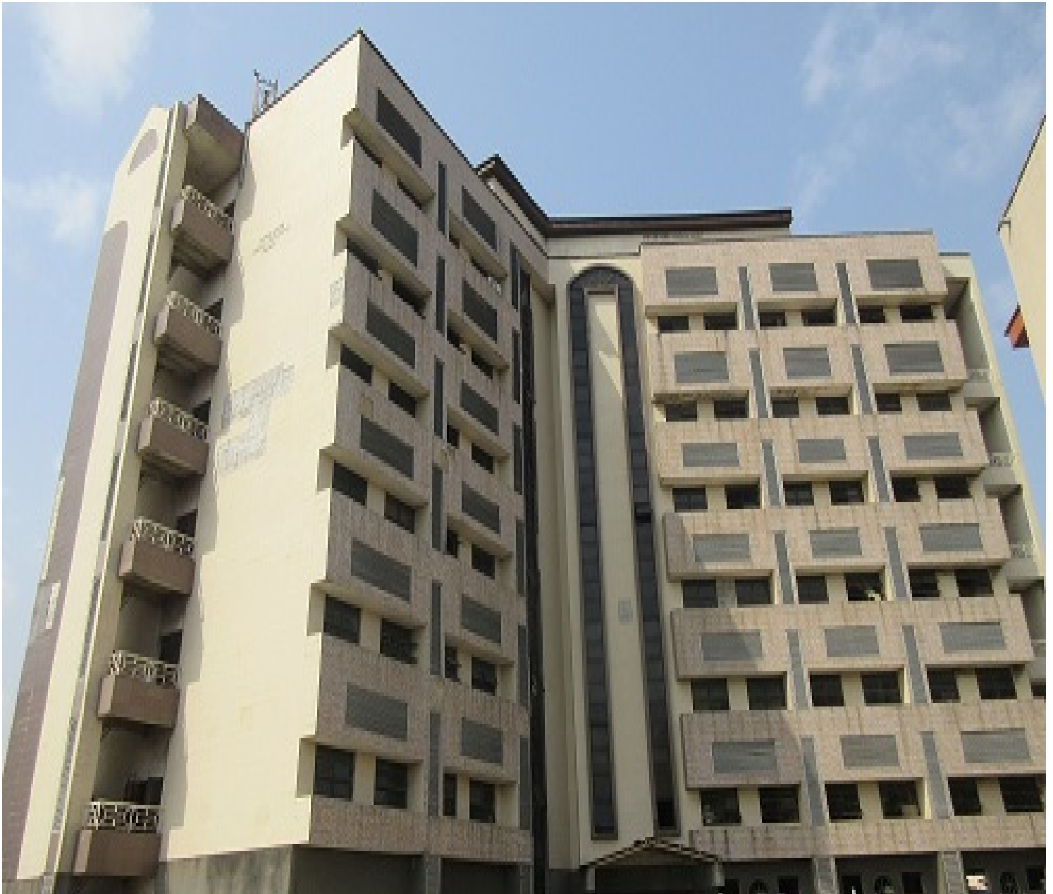
Seven Storey Building, Yaba College of Technology, Yaba, Lagos
