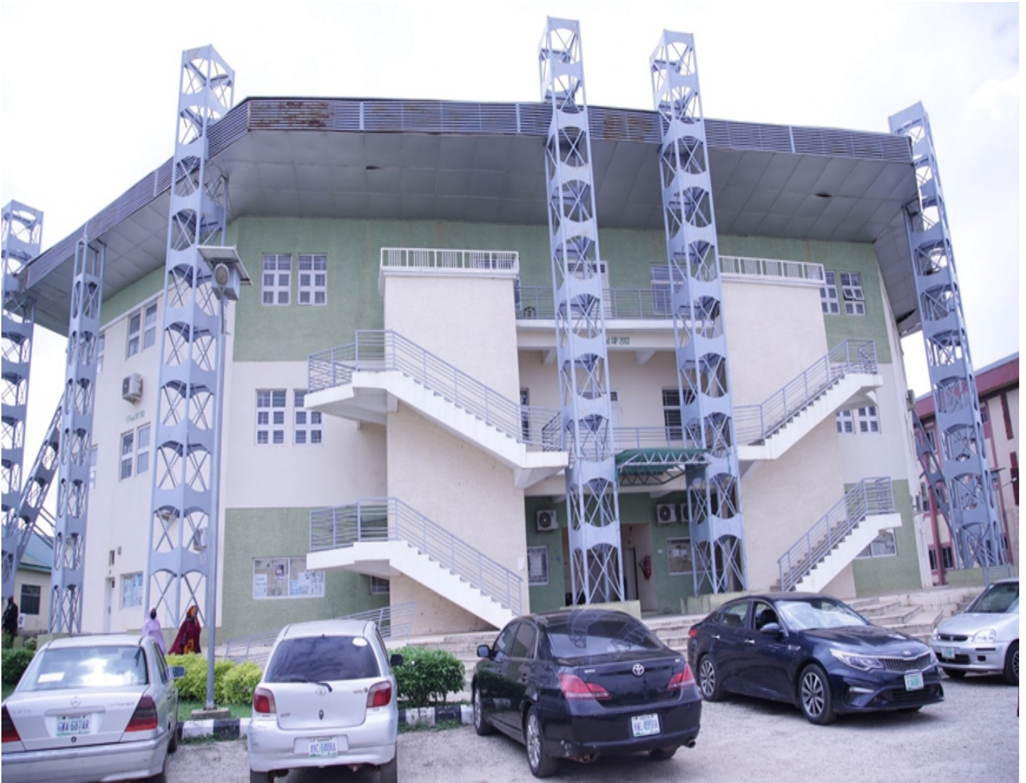
1000 Seater Auditorium, Kaduna State University, Kaduna
