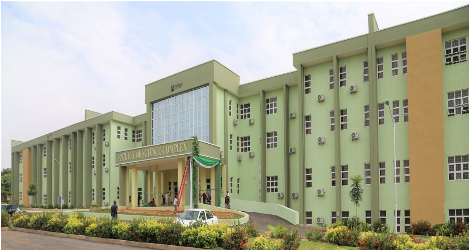
The Faculty of Science Building at Gombe State University
